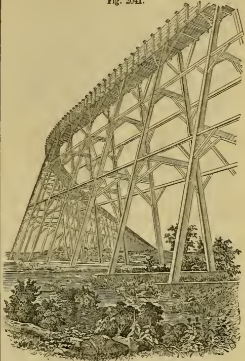
Flume near Smartsville, Yuba County, California.
